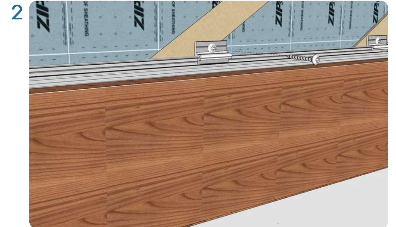
2 Insert siding into the starter strip and apply downward pressure on the board while securing the rain-screen clip, and then fasten the board with the rain-screen clip and screw.
