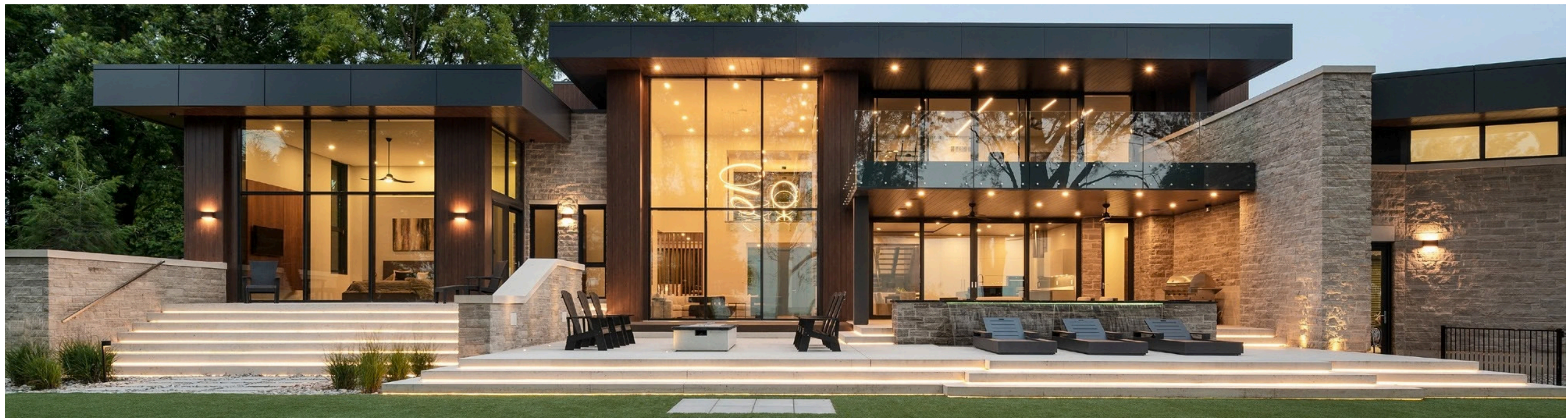
Private Residence, St. Catharines, Ontario John Willmott Architect
